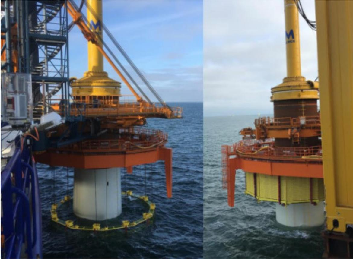
*AdBm noise mitigation system deployed during foundation installation (left) and AdBm system in retracted position, prior to deployment (right)*
